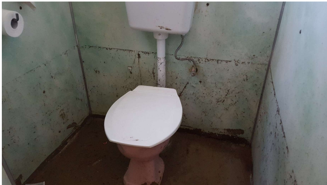
Figure 3-4 Flood Mark Visible at 108 Whyte St
