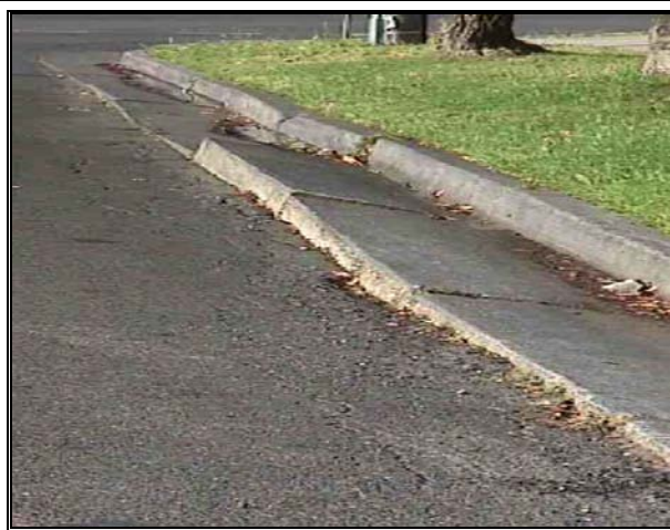
Condition 9 Extreme movement and lack of function
