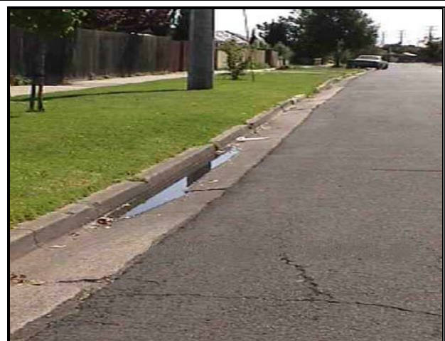
Condition 8 Large movement and holding of water
