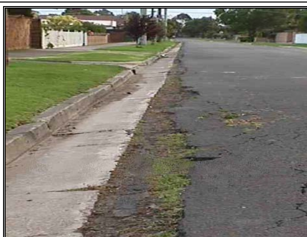
Condition 6 Movement and concrete breakdown
