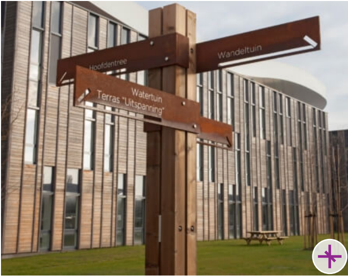
Simple timber and lasercut corten steel directional signage.
