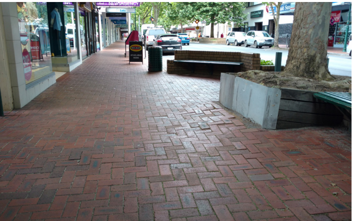
Build outs at pedestrian crossing points defined with seating/planters require updating, including appropriate management of insufficient free growth area.
