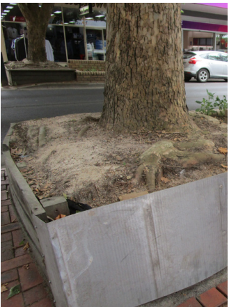
Tree planters are currently deteriorating due to insufficient growth area and require reconsideration.
