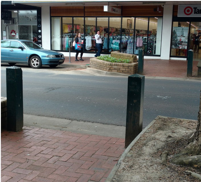
Poor marked crossing prioritises vehicles over pedestrians increasing potential for collision and injuries to occur.
