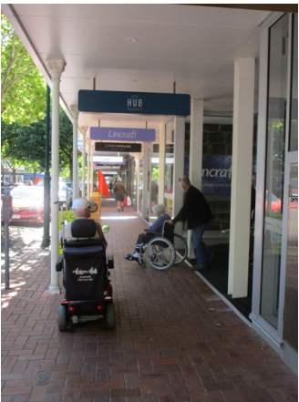
Existing brick pavers currently cause safety concerns due to level issues and surface slipperiness.
