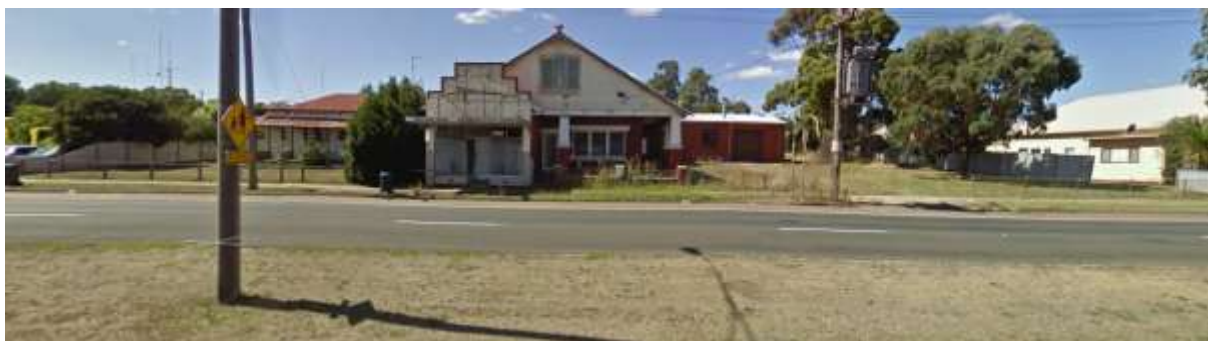
Figure 2 above. Google street view of the frontage of all sites
