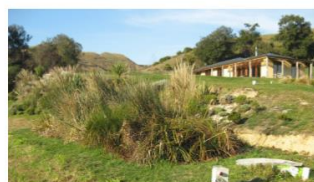
Reed bed – passively treats the wastewater using natural processes as it moves through vegetation.
