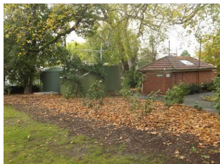
Figure 11: Toilets and water tanks
