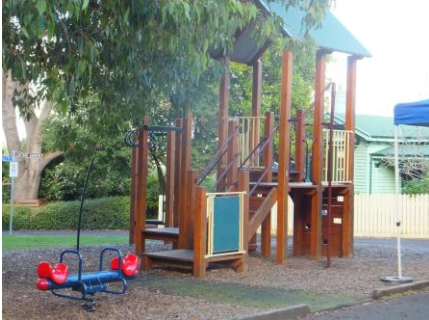
Figure 36: New timber fort and springer
