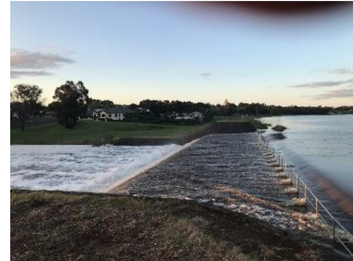
Figure 22: Hamilton weir in flood (early 2021)
