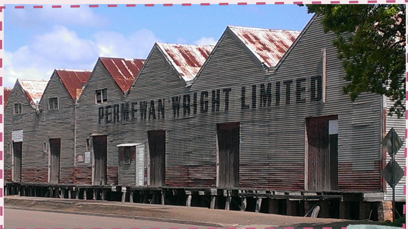
Permewan's Sheds Hamilton – demolished 2018
