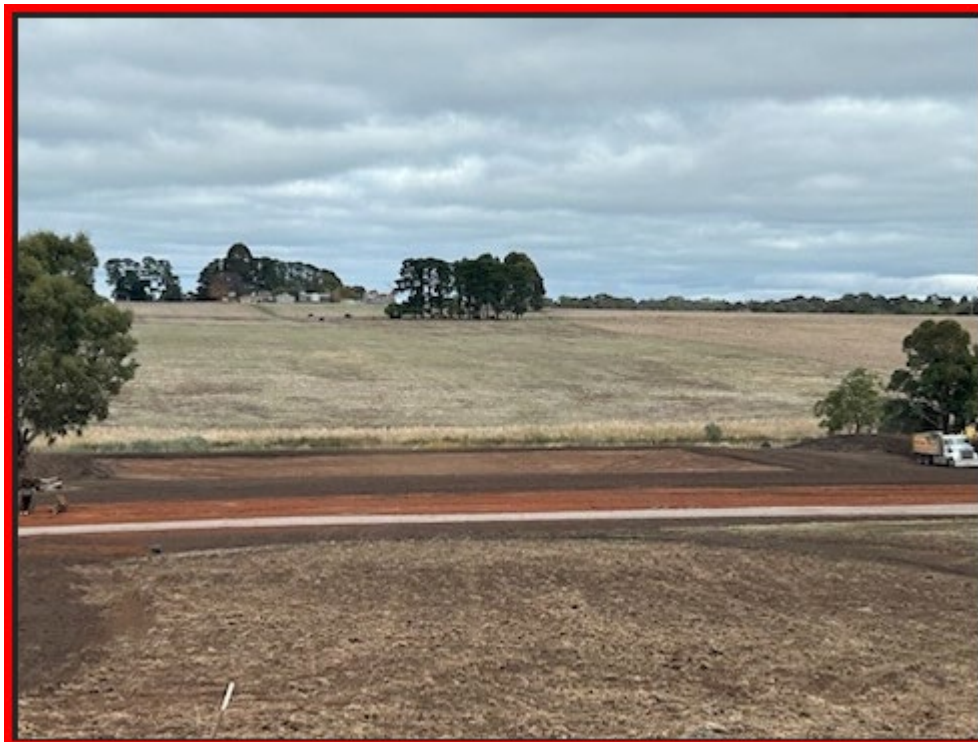
Figure 1: showing earthworks that have commenced at the site.
