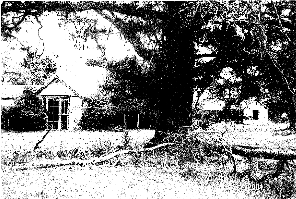
Spring Vale Homestead Complex, Hillview Road, Coojar. Dining Room & former Post Office
