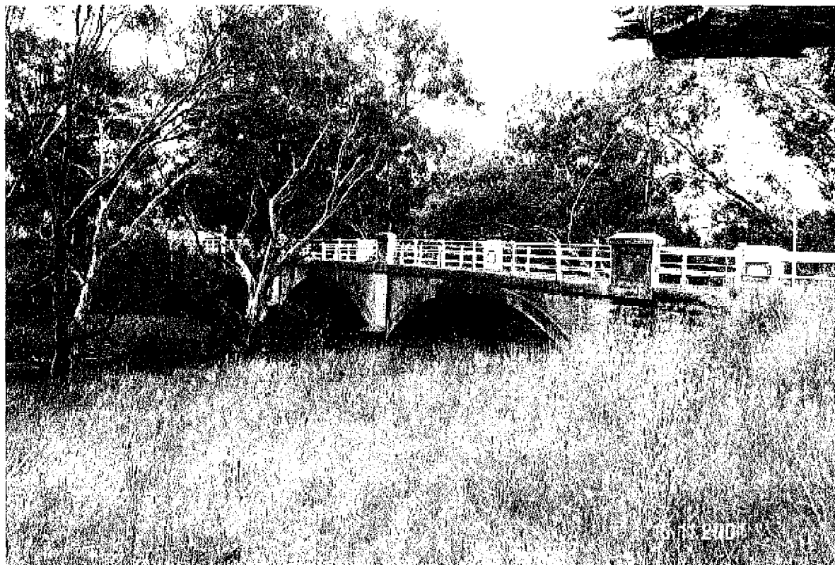
Monier Bridge, Brung Brungle Road, Wannon
