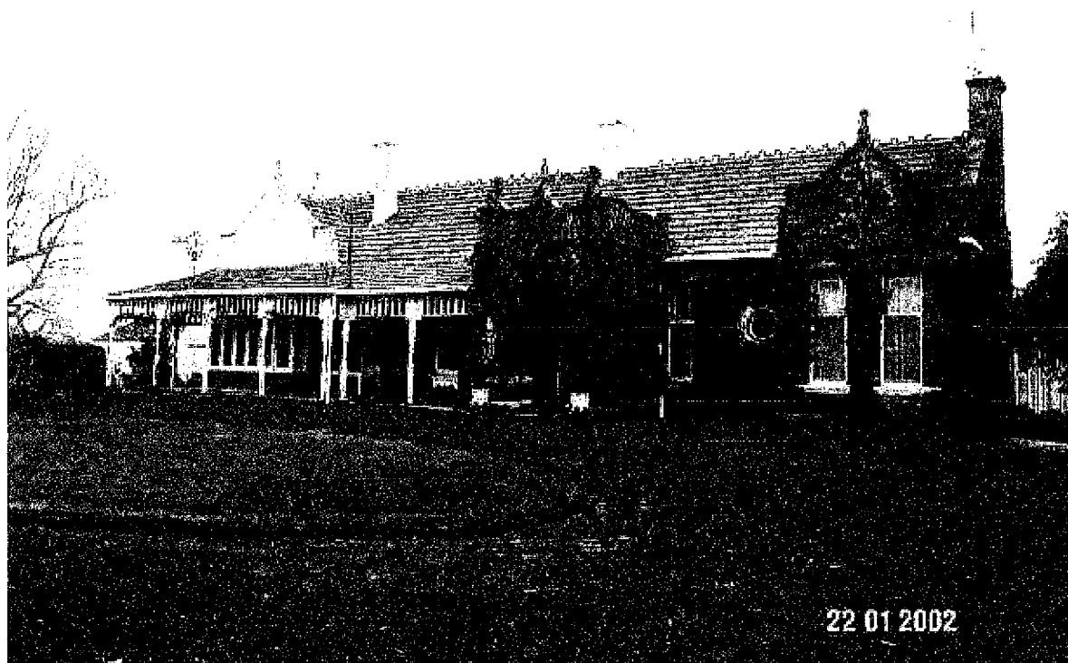
Bassett Homestead, Bassett's Road, Branxholme. Front elevation
