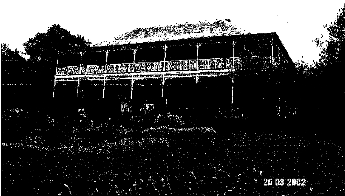
Arrandoovong Homestead Complex, Branxholme. Front Wing of Homestead.
