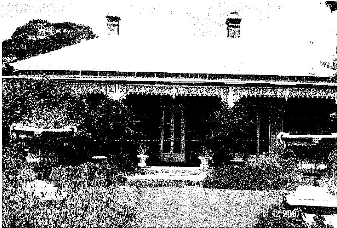
Viladale House Complex, McKellar's Road, Yulecart. Front elevation
