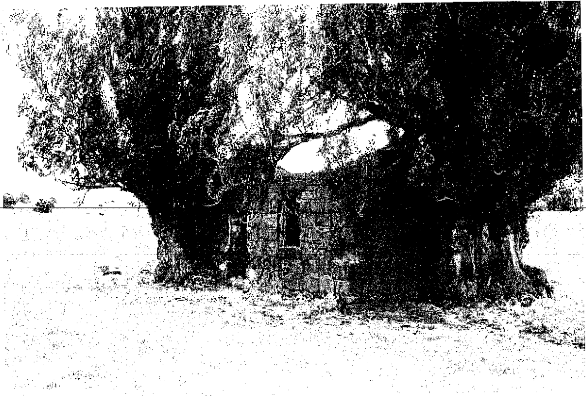
Krummnow's House, Herrnhut, Penshurst
