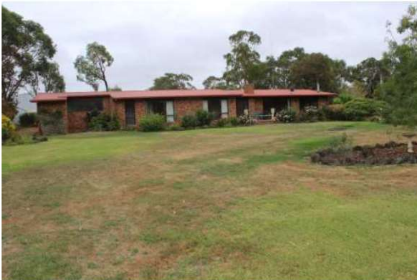
Photograph 6: Rear (east) elevation of existing dwelling
