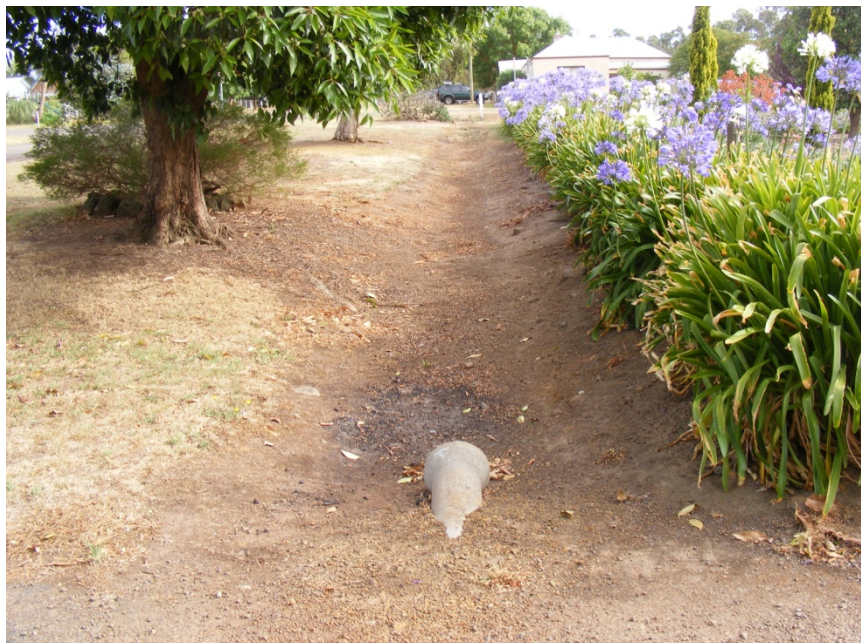
FIGURE 3-9 TYPICAL STORMWATER SWALE/TABLE DRAIN
