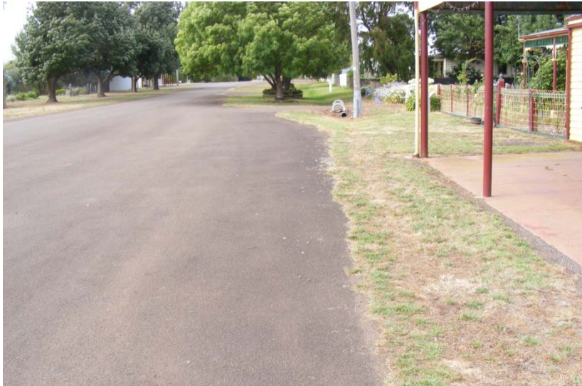
FIGURE 3-8 MCNICHOL ST. SMALL ALLOTMENTS, AND POOR SURFACE WATER DRAINAGE ISSUES
