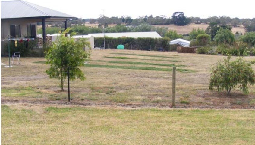
FIGURE 3-5 EXAMPLE OF EVAPO -TRANSPIRATION TRENCHES
