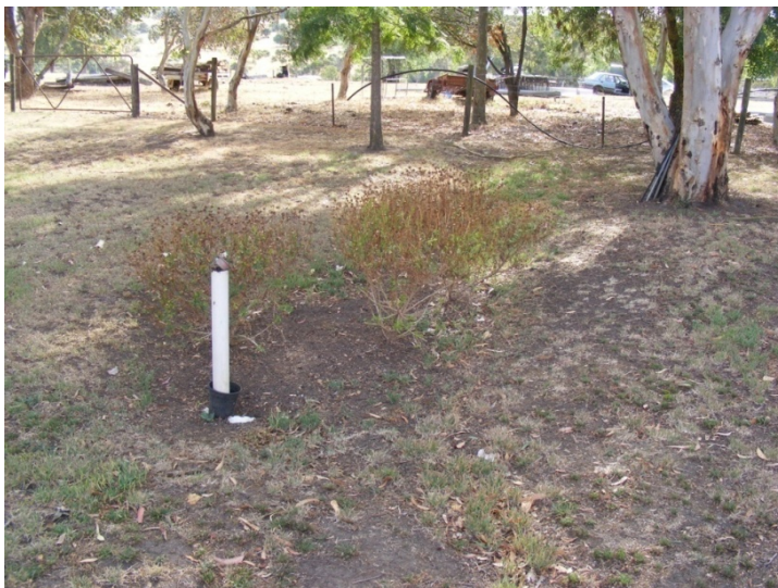
FIGURE 3-4 TYPICAL ABSORPTION TRENCH AND VENT
