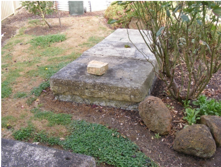
FIGURE 3-3 TYPICAL DOMESTIC BLACKWATER SEPTIC TANK
