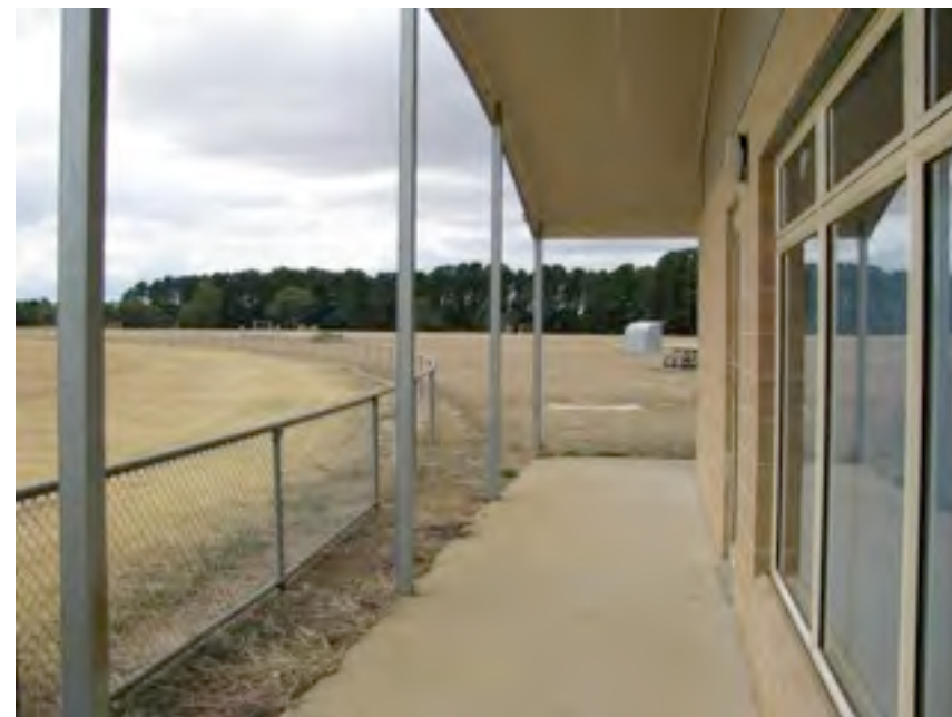
Image 11: Pedrina Park, Ansett Pavilion
