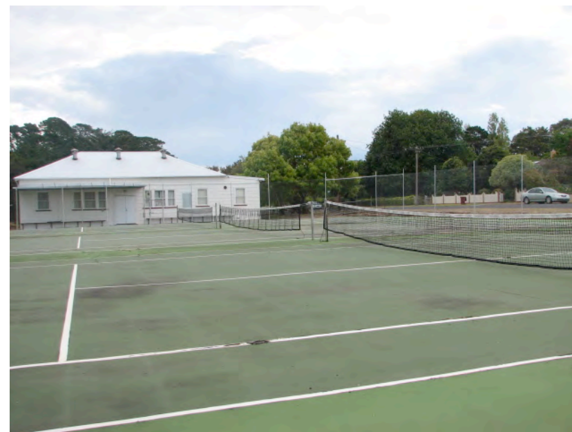
Image 7: Patterson Park, plexipave courts and hall
